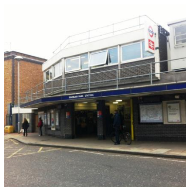
Photo 14: Western station entrance
