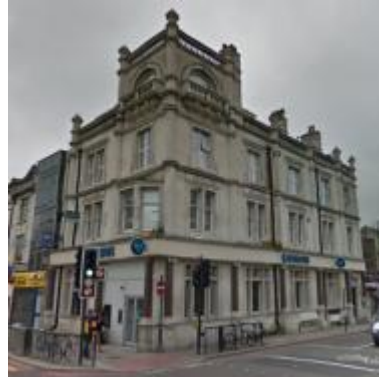
Photo 35: Intact historic fabric
