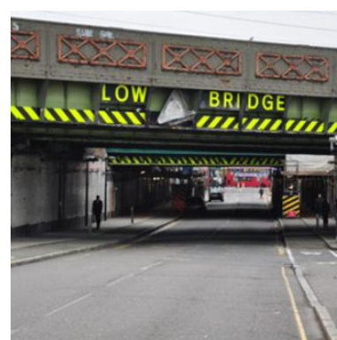
Photo 12: Bridge, Stroud Green Road
