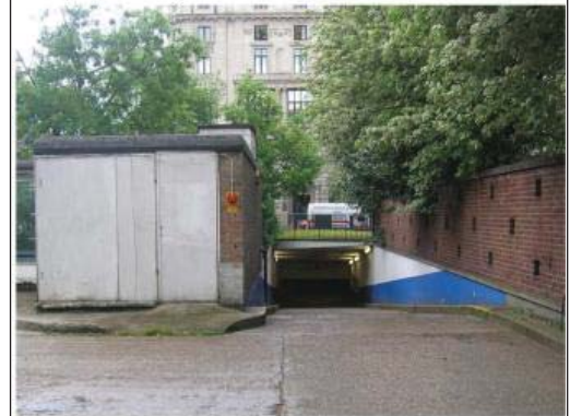
Finsbury Square, carpark ramp
