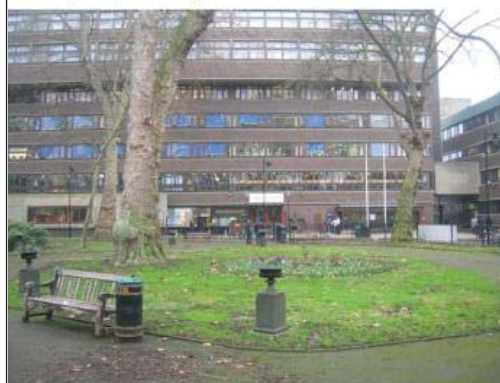
Northampton Square looking north
