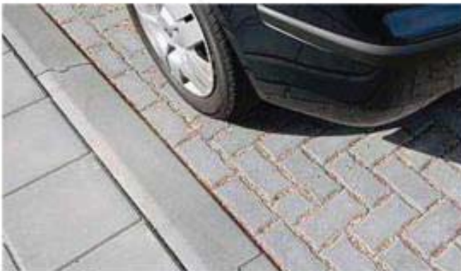
Permeable Paving
