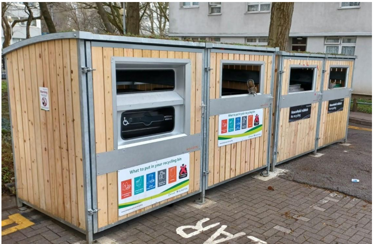
Figure 5 Recycling and refuse bin store, including accessible recycling bin and green roof
